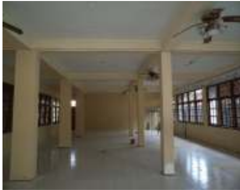
Gambar 4. Rehabilitasi SMAN 3 Banda Aceh
