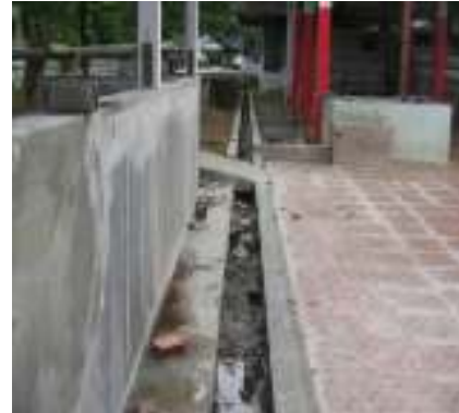
Gambar 51. Rehabilitasi prasarana RPH
