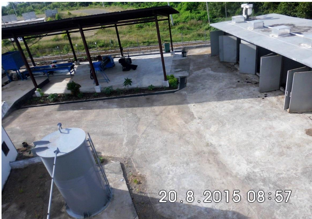
Gambar 3.55 Intermediate Treatment Facility di TPA Gampong Jawa
